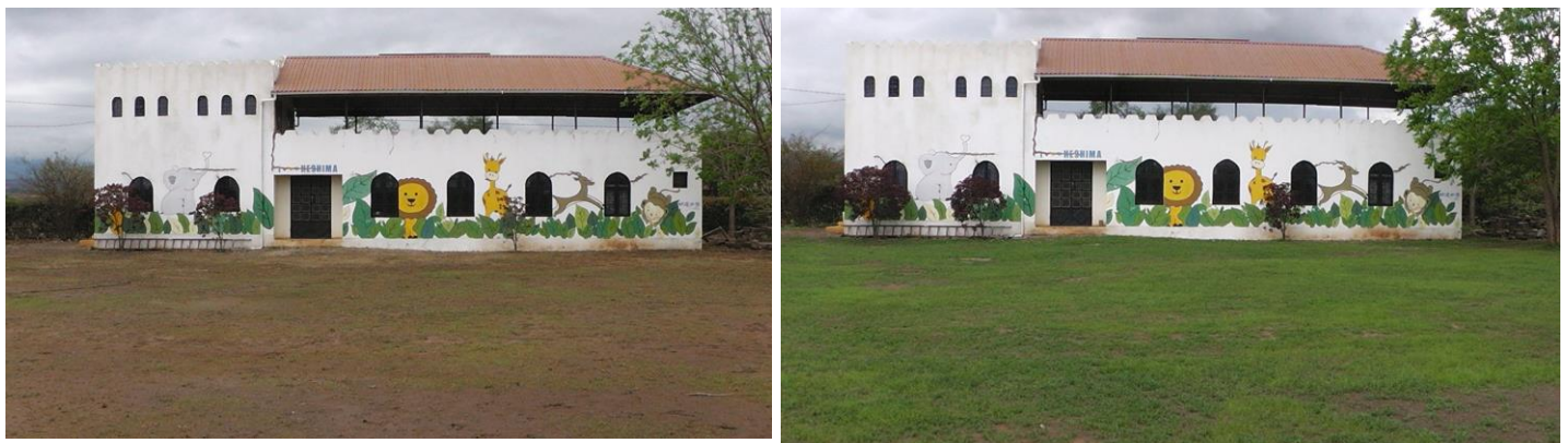
Photos show Heshima before and 2 days after the rain started
